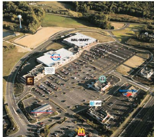
Grading has commenced on the 4.3 acres for 2 nd Q 2011 Delivery
